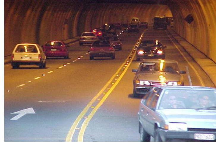
Terrace Tunnel (Wellington, NZ)
